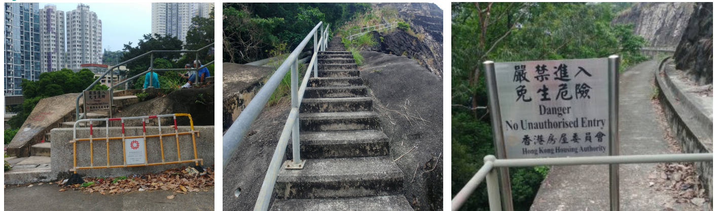
Figure 41: Unauthorised use of maintenance tracks in Shau Kei Wan
