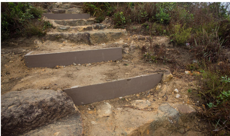
Figure 48: Wood/plastic composite boards with soil backfill
