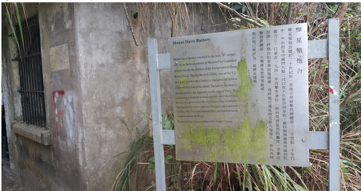
Figure 21: Corroded interpretive panel on Mount Davis
