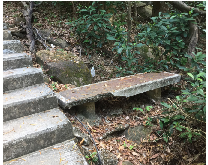
Figure 82: Seating in poor condition on Fu Yung Shan
