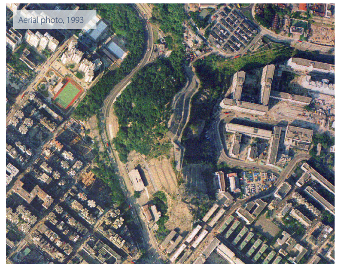
Figure 7: Construction of Shek Kip Mei Service Reservoirs No. 2 and No. 3, 1993-2000
